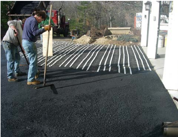
Asphalt being compressed over ClearZone snowmelt system.
