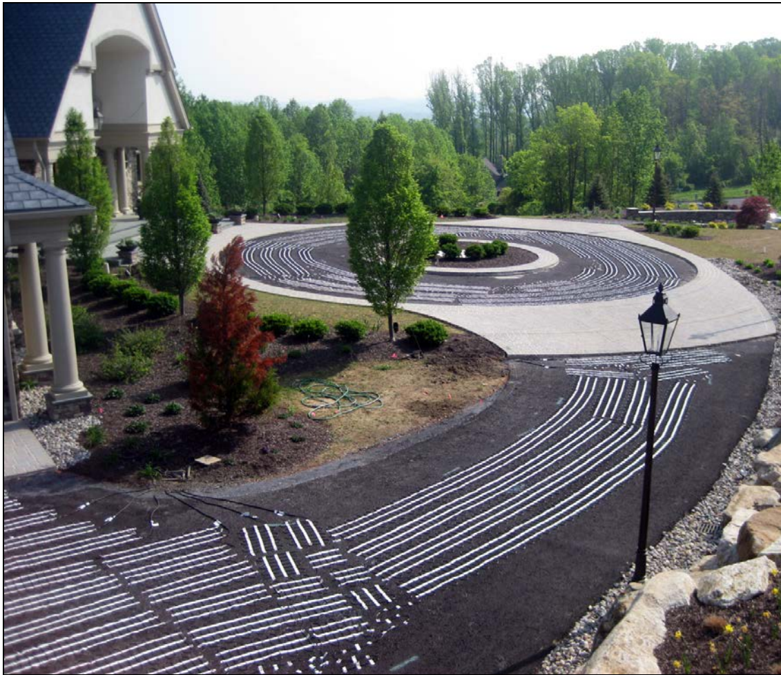
ClearZone heated asphalt and paver driveway being installed.
