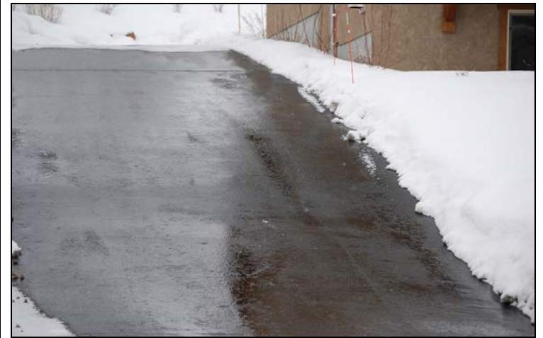
ClearZone asphalt heated drive and parking ramp.
