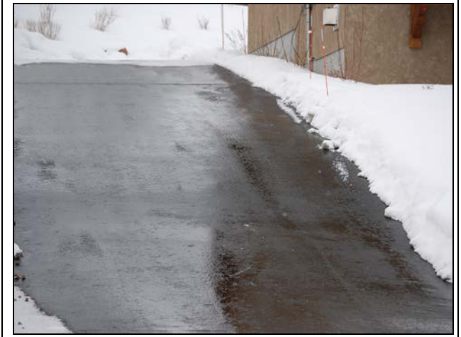
Commercial heated asphalt ramp to parking area.
