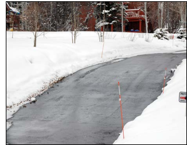
ClearZone heated asphalt driveway.
