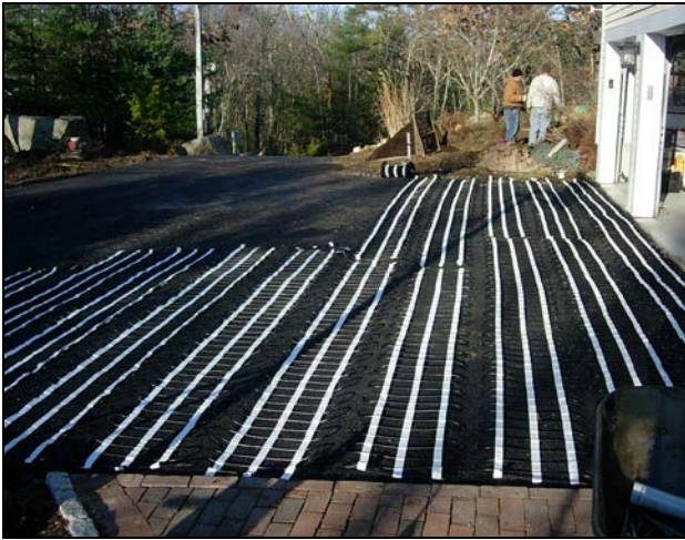
ClearZone snow melting mats being installed for heated asphalt driveway.
