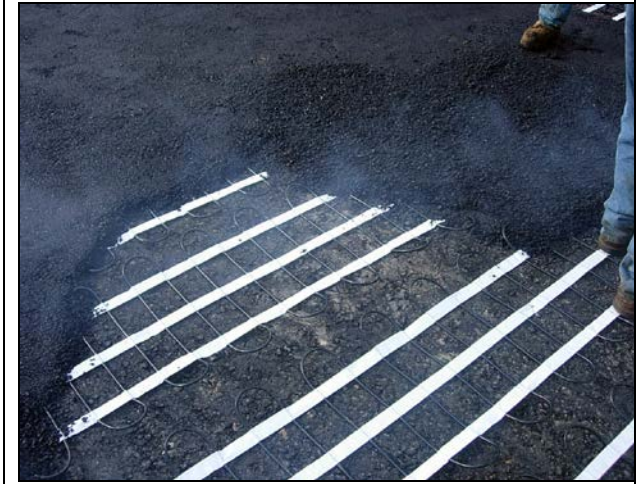
CZ snow melting cable and mats are designed to withstand the extreme temperature of hot asphalt applications.
