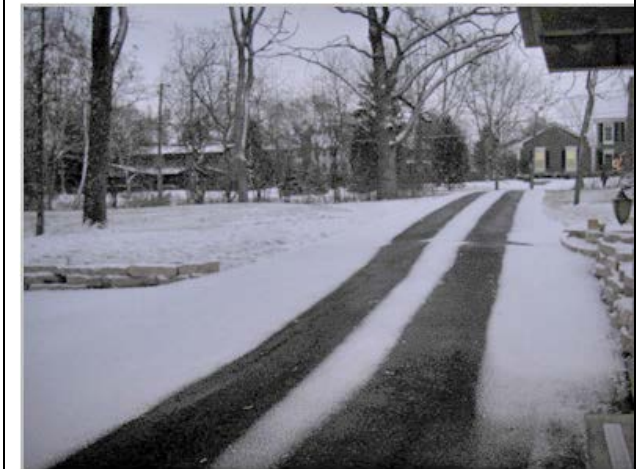
AFTER: Completed asphalt tire track heated driveway.
