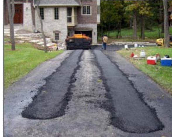
Asphalt applied over the CZ mats.
