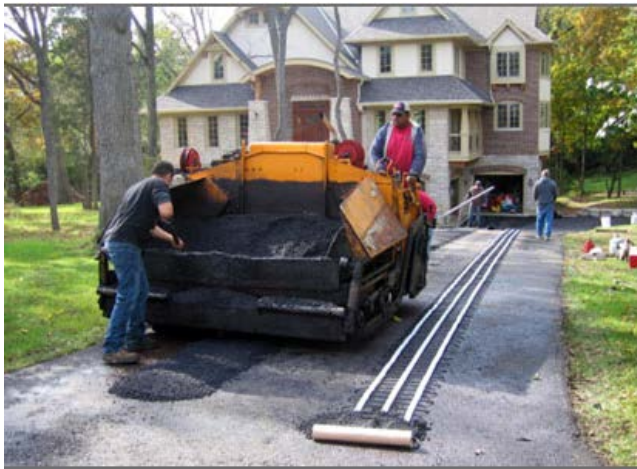
BEFORE: ClearZone mat rolled out for heated tire asphalt tracks.
