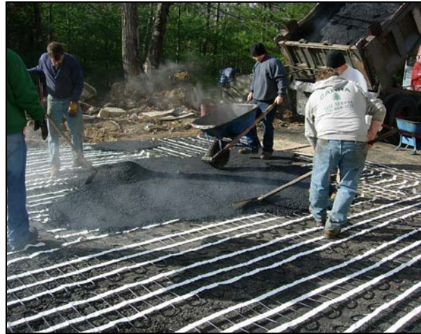
Hot asphalt being applied over ClearZone snow melting mats.
