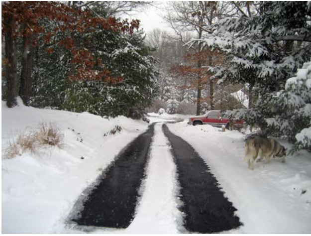
ClearZone heated asphalt tire track driveway.
