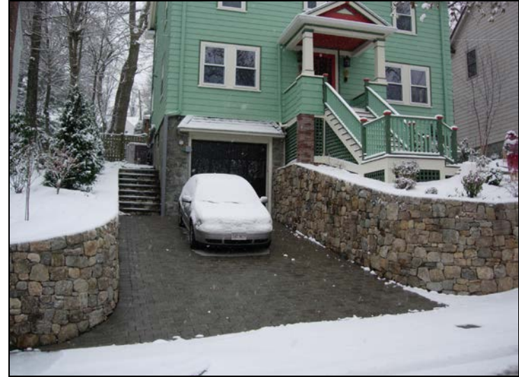
AFTER: Warmzone paver heated driveway in operation.
