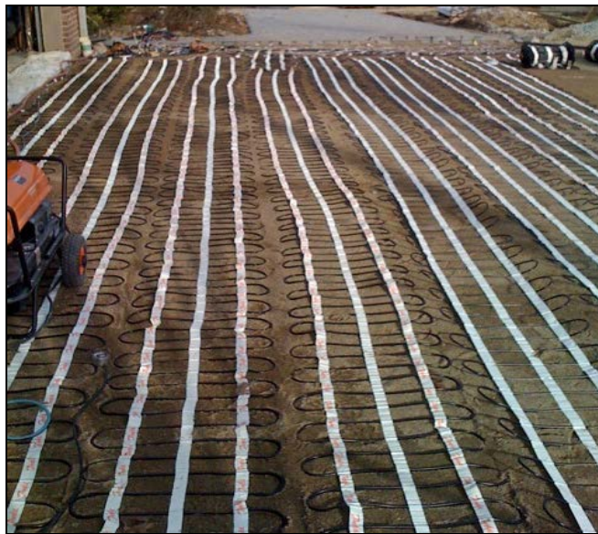
BEFORE: ClearZone snow melting mats being installed.
