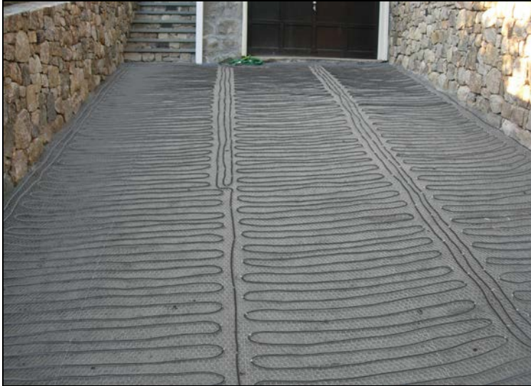
BEFORE: ClearZone heat cable being installed under paver driveway.
