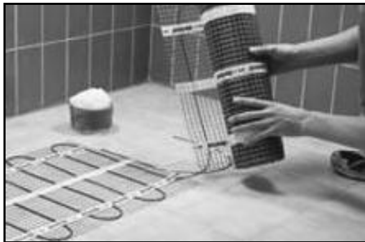
Figure 2: Cut mesh backing to turn the heating mat for the desired layout.
