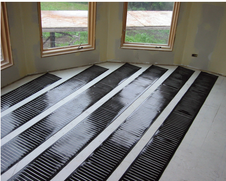
The FloorHeat STEP heating element is easy to install and features maintenance free operation.
