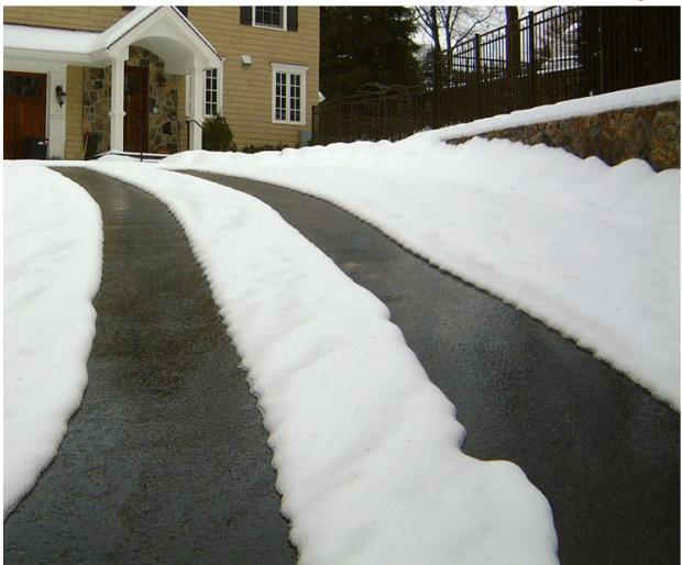
Heated tire tracks in asphalt driveway.
