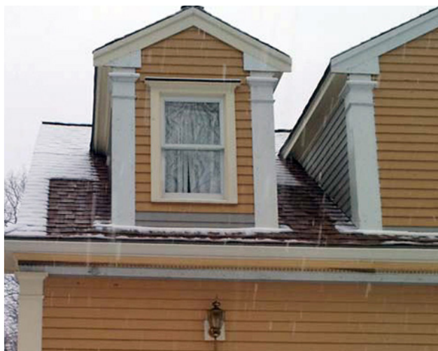
Roof deicing system heating roof edges.
