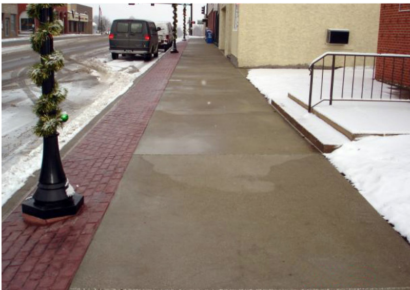
Warmzone heat cable embedded in city sidewalks.
