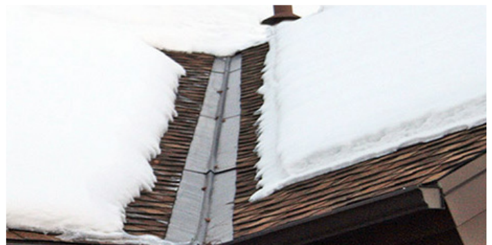
Warmzone RoofHeat STEP low-voltage roof deicing system heating roof valley and edges.
