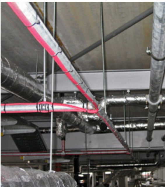
Pipe tracing system installed.
