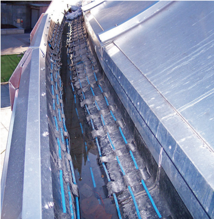
Warmzone roof deicing heat cable installed in commercial gutter melt application.
