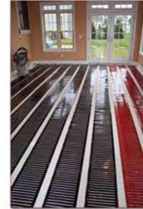
Installing a low-voltage radiant floor heating system.
