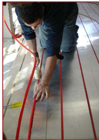
PEX tubing being installed in Raupanel for Warmzone hydronic floor heating system.
