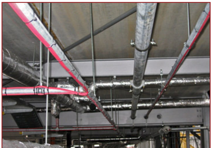
Industrial pipe tracing application.
