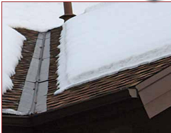
Warmzone low-voltage roof heating element installed in roof valley.
