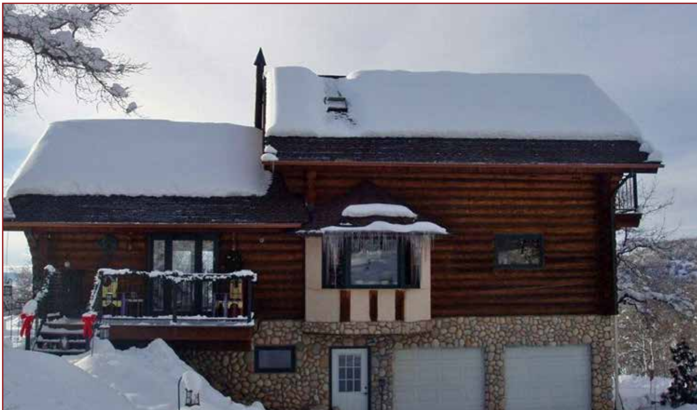
Mountain cabin with low-voltage roof deicing system installed at the roof edges.
