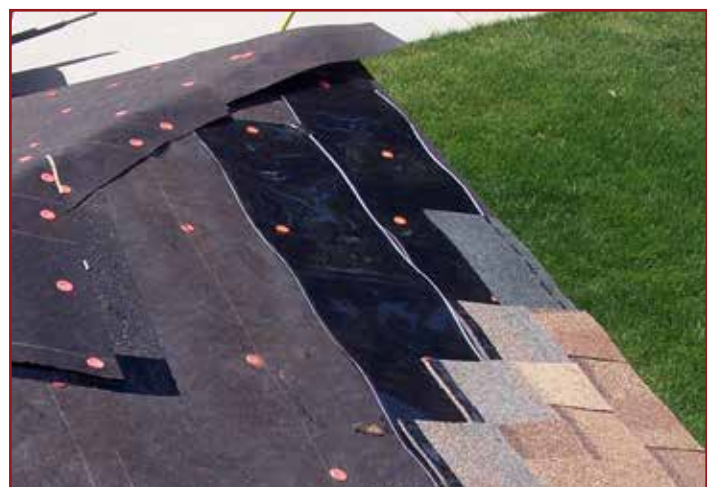
Heating element being installed under shingles.
