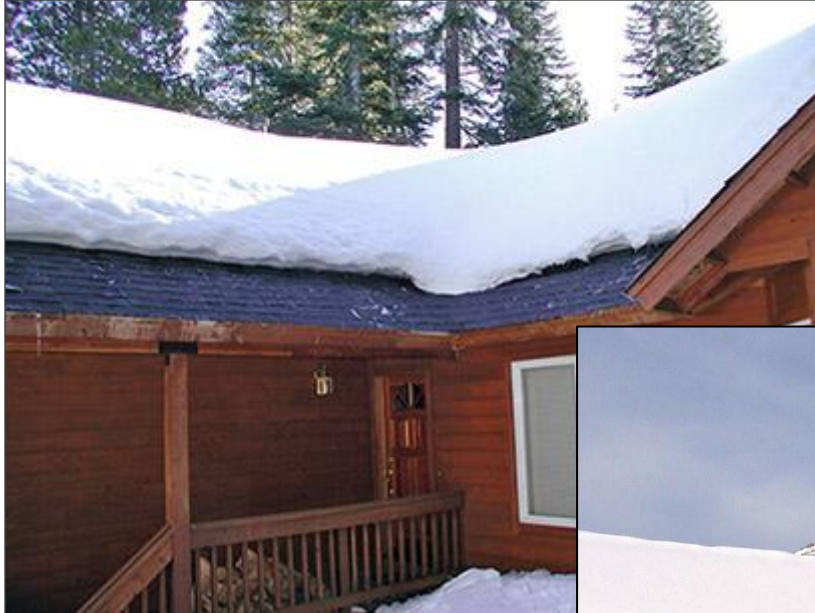
Heated roof edges and valleys.
