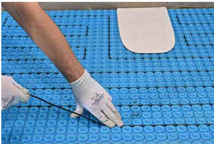
ComfortTile heat cable being installed in the channels of the Prodeso membrane.
