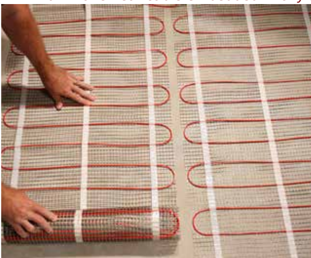
Installing floor heating mats.
