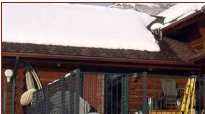
Heated roof valley and edges.
