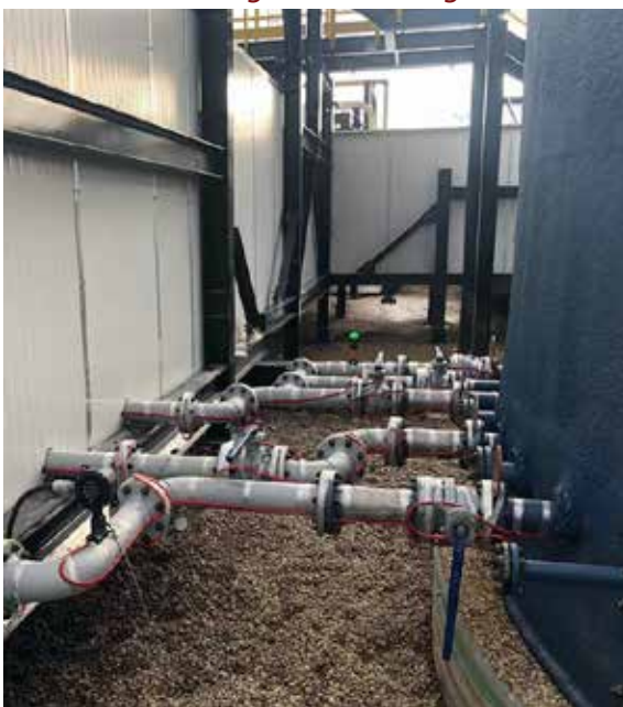
Pipe tracing system installed.
