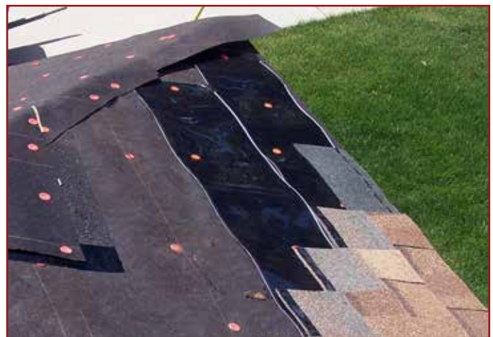
Heating element being installed under shingles.
