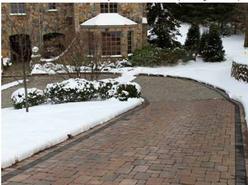
Warmzone snow melting system installed in paver driveway.
