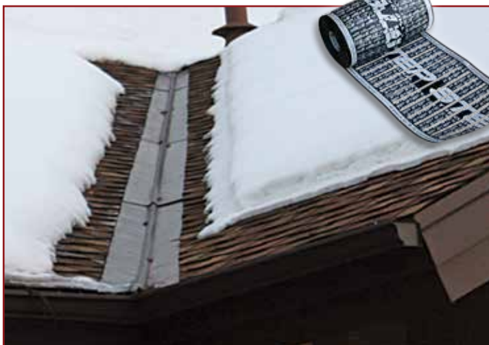
Warmzone low-voltage roof heating element installed in roof valley.
