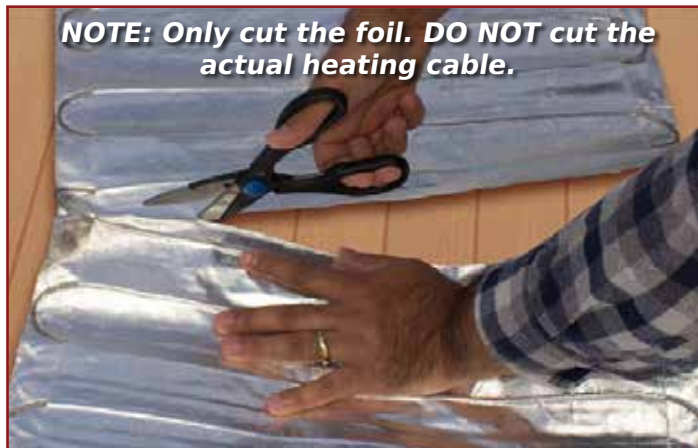
FoilHeat mats can be easily cut on site. (Depending on your heating requirement, FoilHeat is available in 120 and 240 volts at 12 watts per square feet.)
