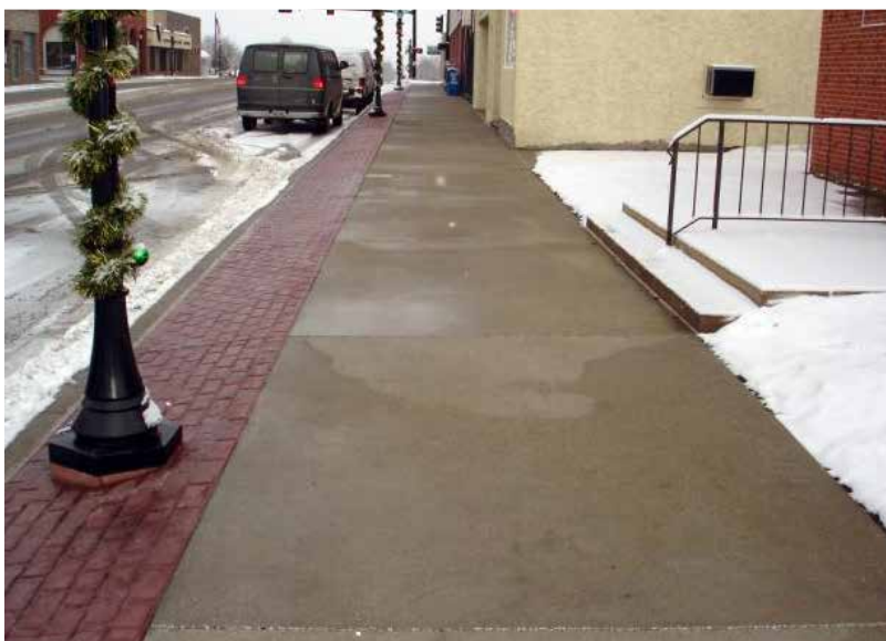
Warmzone heat cable embedded in city sidewalks.
