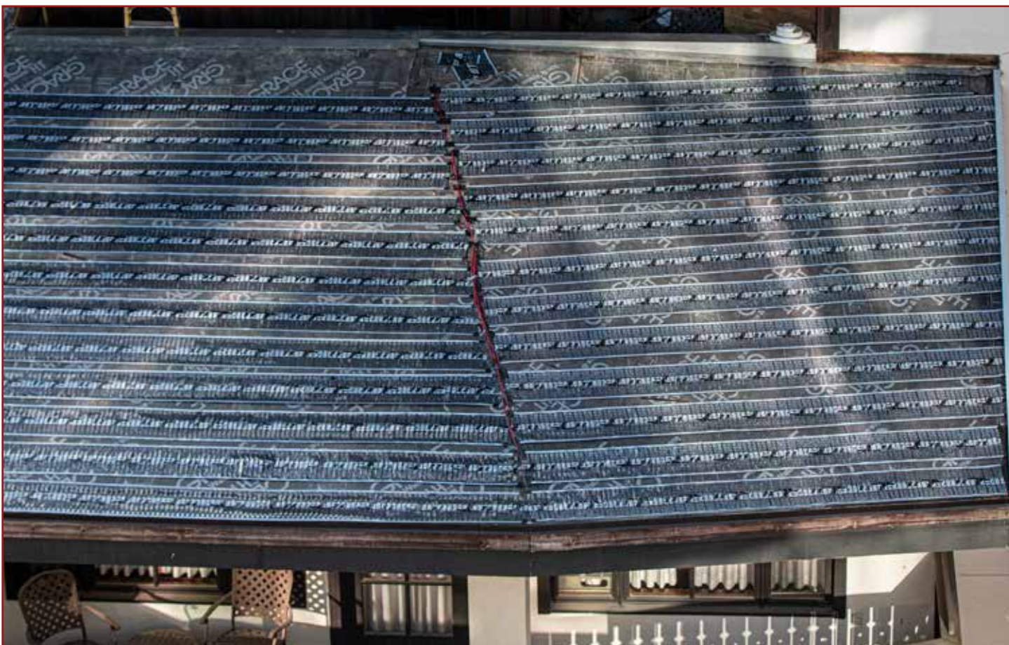
Resort hotel with low-voltage roof deicing system being installed.
