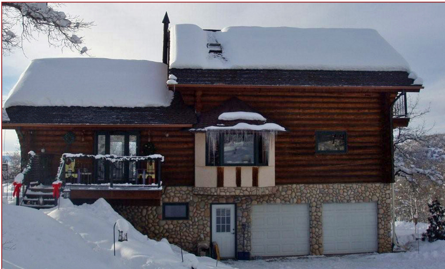
Mountain cabin with low-voltage roof deicing system installed at the roof edges.
