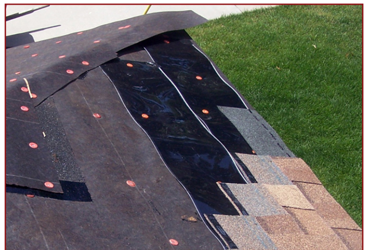
Heating element being installed under shingles.
