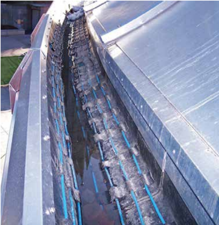
Warmzone roof deicing heat cable installed in commercial gutter trace application.
