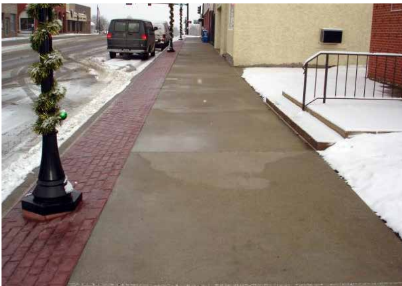
Warmzone heat cable embedded in city sidewalks.
