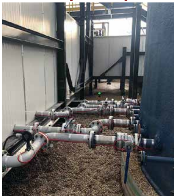
Pipe tracing system installed.
