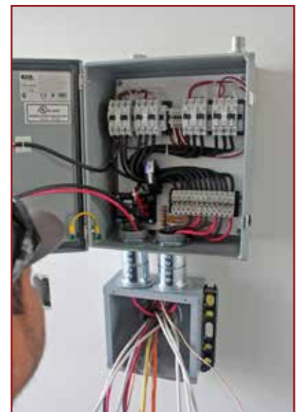
Contactor panel being installed.
