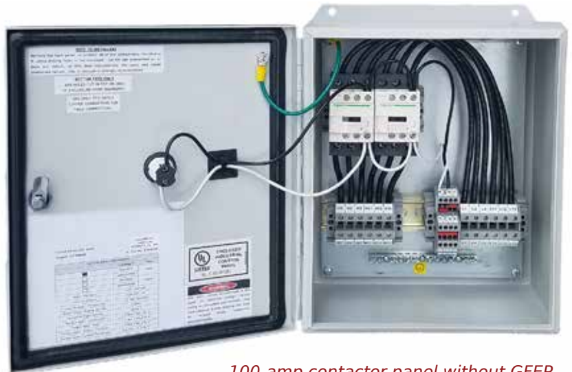
100-amp contactor panel without GFEP (two 50-amp contactors).
