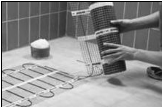
Figure 1: Cut mesh backing to turn the heating mat for the desired layout.
