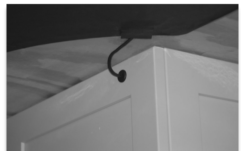
Cable hole after finishing plug is installed.
