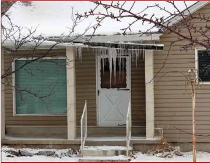
Above: Example of gutter damage caused by heavy ice buildup. Right: House with roof deicing system installed at roof's edge.
