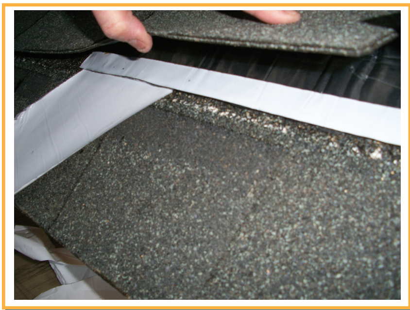
Figure 11. Removing Release Liner
