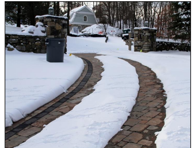
Heated paver tire track driveway
