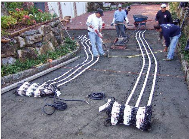
ClearZone snow melting mats being installed for heated paver tire track driveway.
