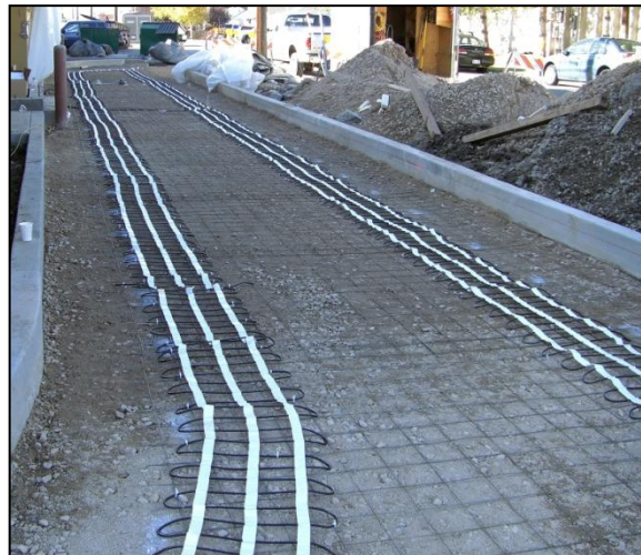
Heated tire track driveway being installed.
